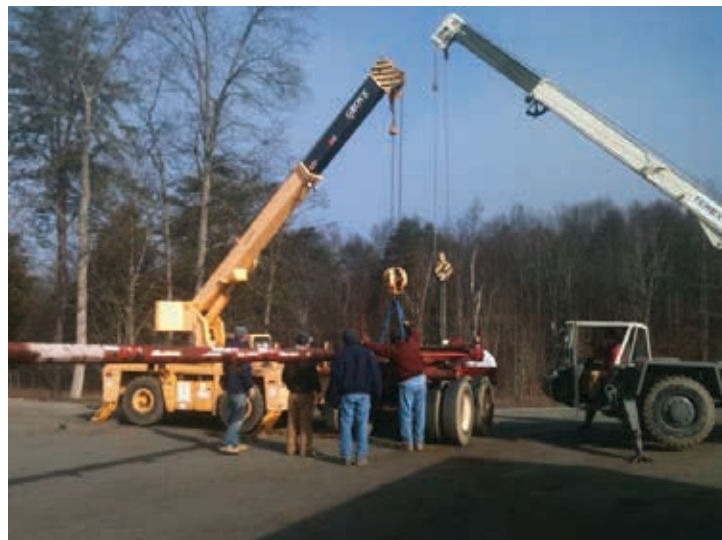
Boston Apprentices loading pipe trailer after Vacuworxs Class wrapped up
