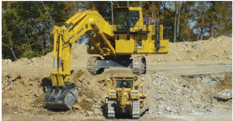
Kokosing Highway project in Pikeville, Kentucky
