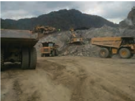
Hi-View highway work in Elkhorn City, Kentucky
